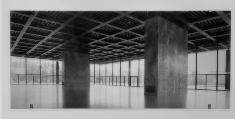
Fig. 2: National Gallery, Ventilation Shafts, 2017
